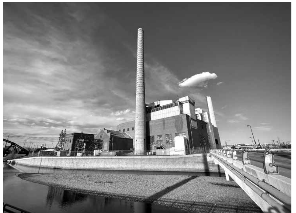
The Zuni Steam Plant has towered over the South Platte River — and the La Alma Lincoln Park, Sun Valley, and West Colfax neighborhoods — since 1901.
