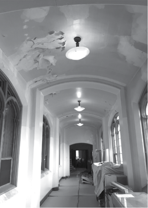
Deterioration of the plaster and windows in the hallway at Miller Center.
